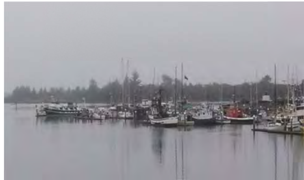
Marinas, piers, wharfs mooring, training walls and breakwaters are overwater structures that tend to result in discrete impacts to eelgrass.
