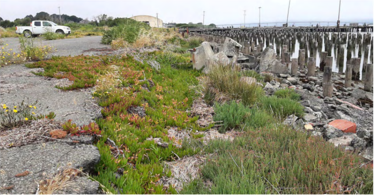
Photograph 25: An example of Estuarine Intertidal Shoreline with saltmarsh vegetation within armored shoreline, east of TP71, looking north. Note MHHW demarked roughly by the wrack line between the saltmarsh vegetation and upland ruderal vegetation. Photograph taken July 8, 2022.
