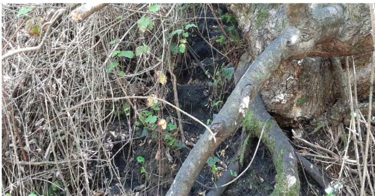
Photograph 39: Typical vegetation for OF18, a two-parameter feature (hydrophytic vegetation and hydrology), taken near TP84 on May 19, 2022. Note black fly ash on soil surface.
