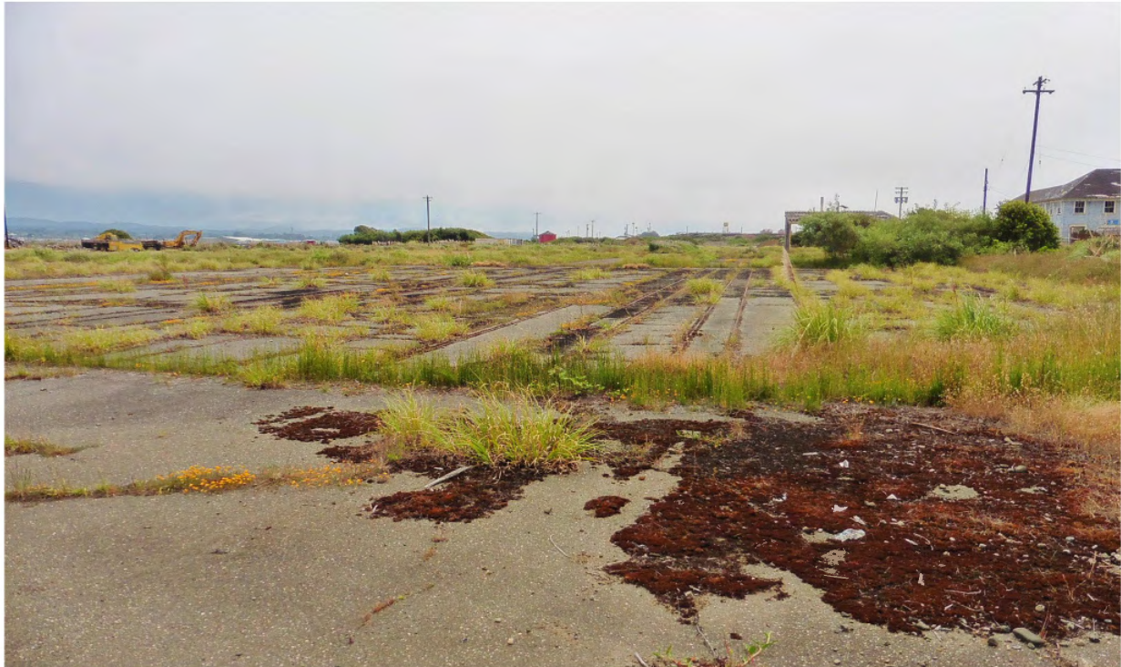
Photograph 17: Artificial aquatic feature- abandoned drying shed foundations beginning to incorporate three parameters. Photograph taken May 28, 2020.
