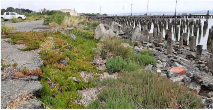
Photo 51: Pickleweed mat at R12, looking north. Note pickleweed mat is restricted to a narrow band of elevation closely associated with the MHHW (located at wrack line) and hardened shoreline with concrete rubble that extends up to asphalt. Ruderal vegetation abuts pickleweed mat. Photo taken August 2, 2022.
