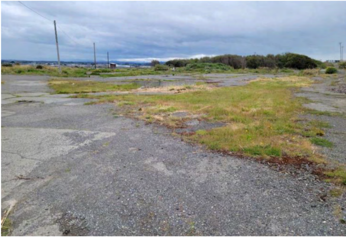
Photo 9: Decaying asphalt with ruderal vegetation looking southeast, typical in large portions of the study area. Photo taken May 6, 2022.
