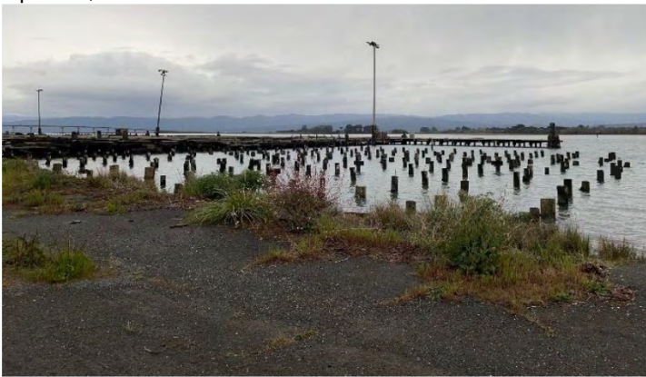
Photo 5: Coastline conditions within the study area looking northeast. Note piles and osprey nests on light poles on existing dock. Photo taken April 13, 2022.
