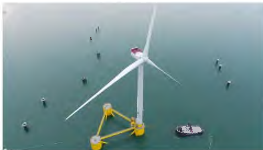
Figure 9: Fixed mooring example (source: Statkraft/KOWL).
