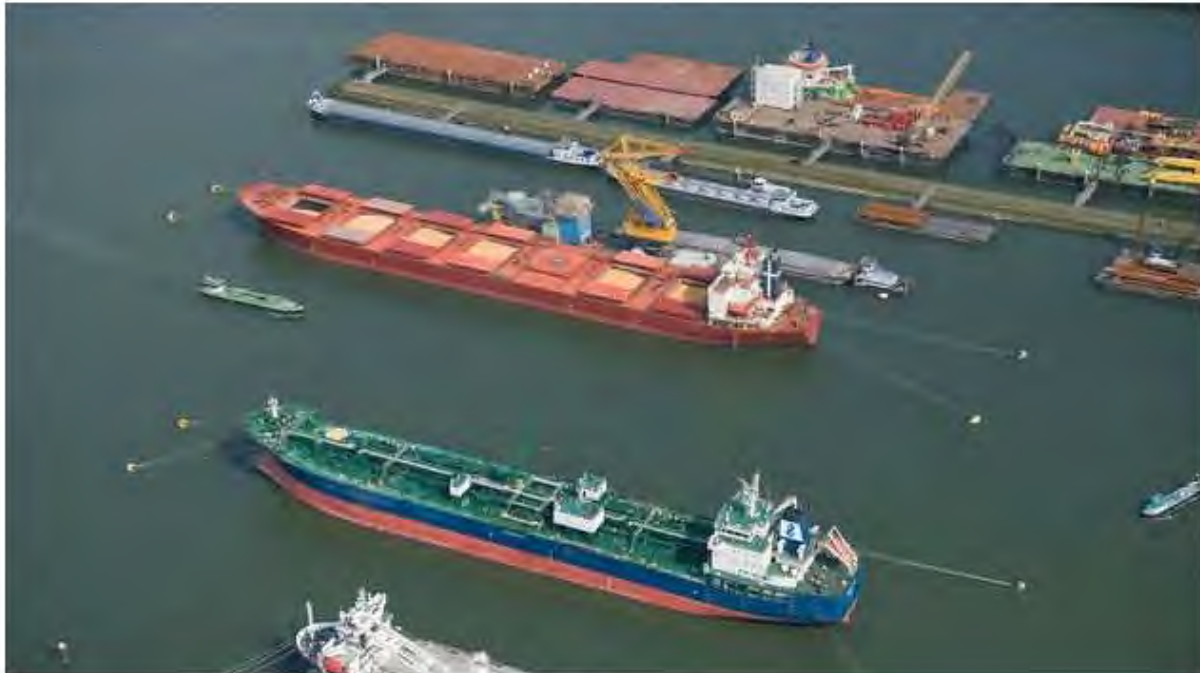
Figure 5: Multi-point mooring buoy example (source: https://www.portofrotterdam.com/en/sea-shipping/buoys-and-dolphins ).
