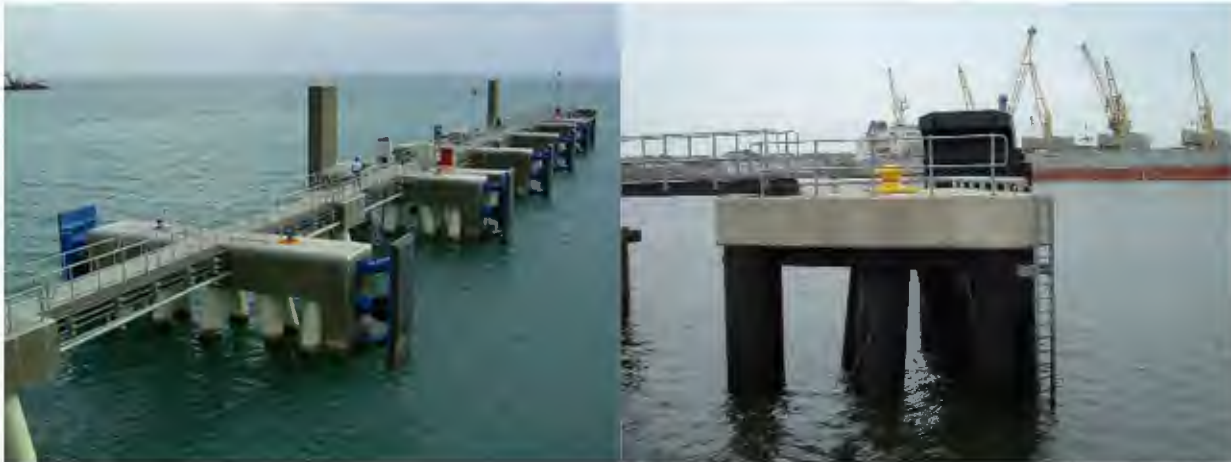
Figure 10: Examples of breasting and mooring dolphins.
