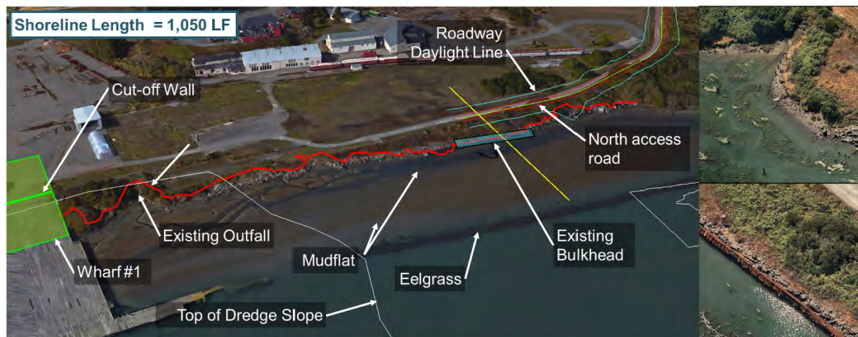
Figure 2-2. Existing Conditions - Reach 1
