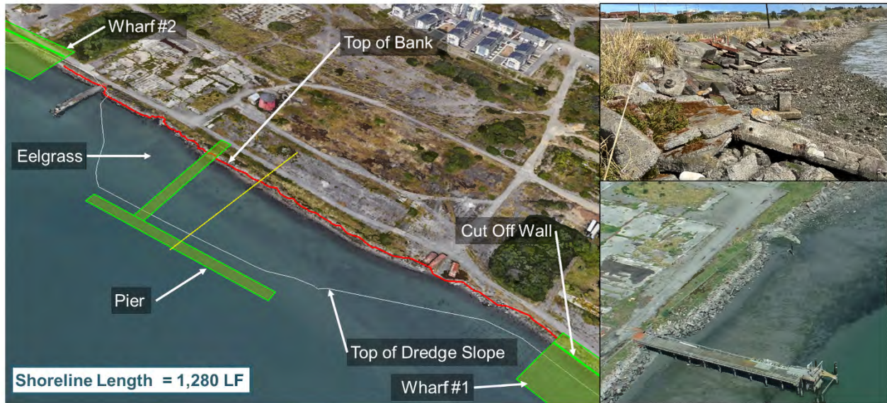
Figure 2-3. Existing Conditions - Reach 2
