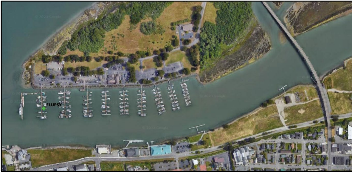
Figure 2. Location of existing floating upwelling system at Woodley Island Marine, Eureka, California.
