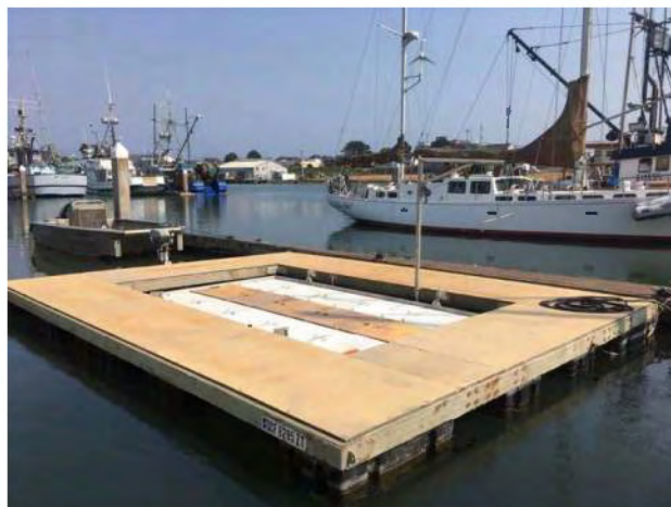
Figure 3. HBOC's floating upwelling system operated at Woodley Island Marina, Eureka, CA.
