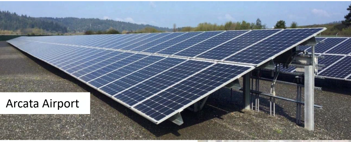
Elevation view of solar array support structure; vertical steel micropiles
