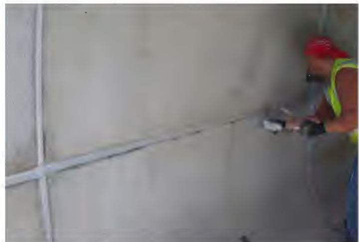
Sealing the interior joints to make the system water-tight
