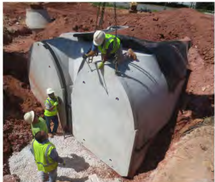
Installation of a typical endwall panel
