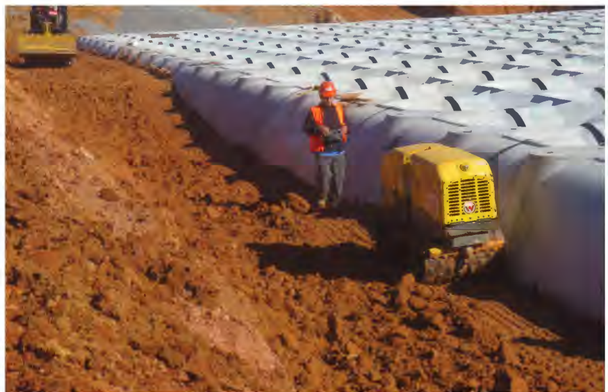
Backfilling structure with on-site soils
