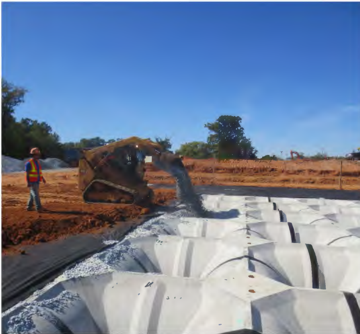
Filling exterior aquifer with stone
