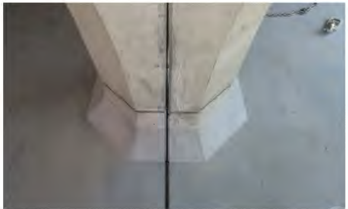
Typical joint between modules
