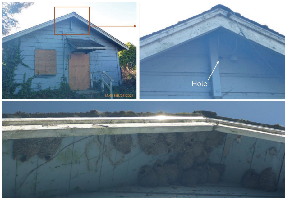
Figure D-6. Area 1 blue shed view from the east side (top left) with access hole to the attic (top right) and prior years barn swallow nests (bottom).
