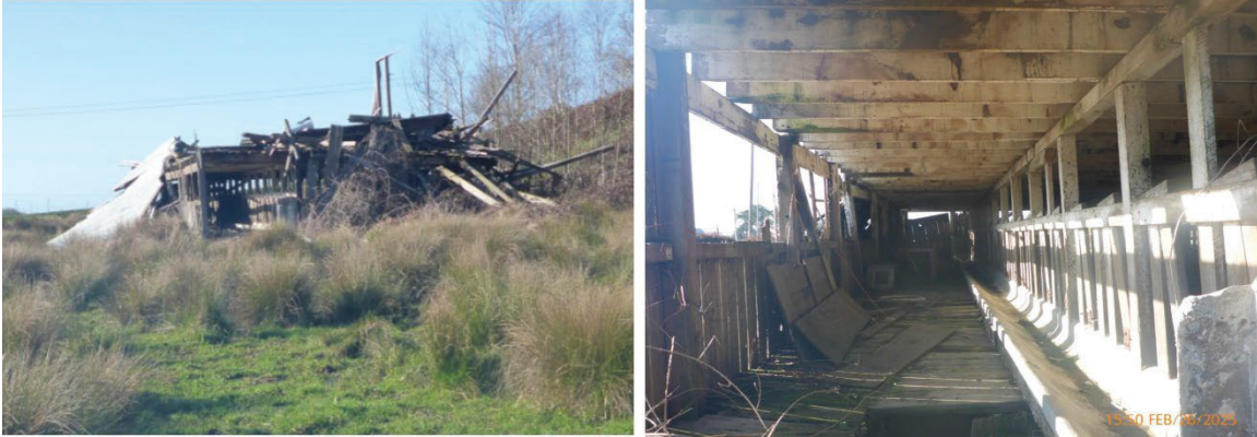
Figure D-11. Area 3 barn and view from the exterior (left) and interior (right).
