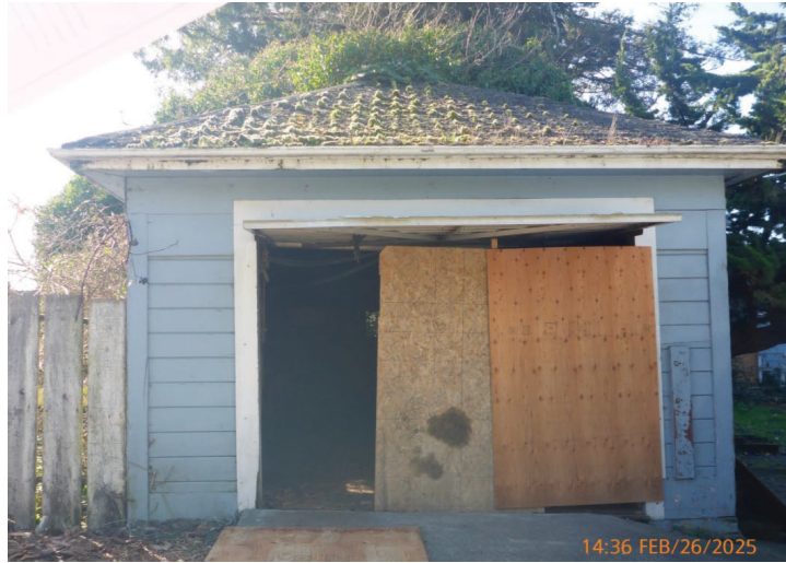
Figure D-7. Exterior view of the Area 1 garage structure.
