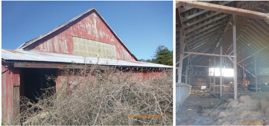
Figure D-4. View of Area 1 barn's southerly exposed exterior (left) and view of the barn interior (right).
