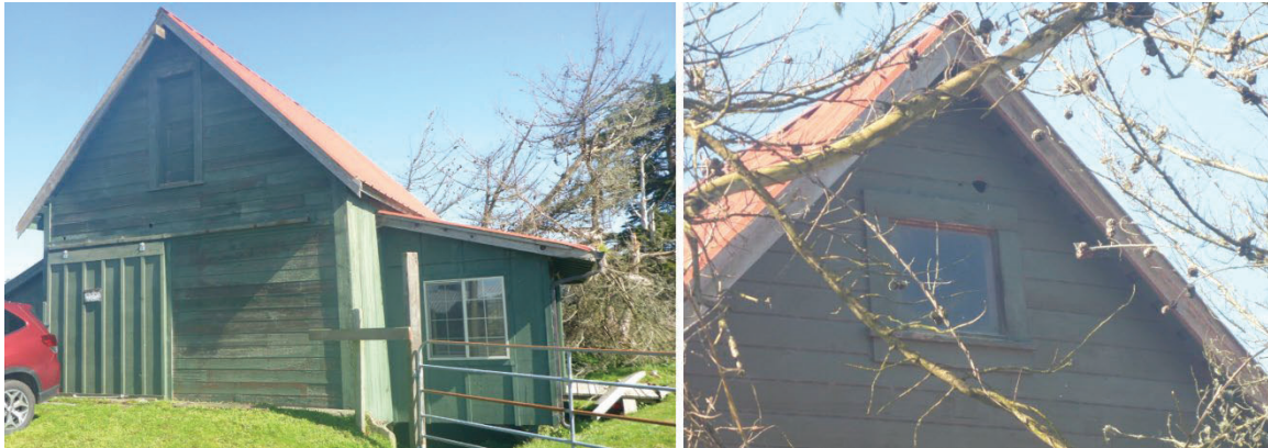
Figure D-12. Area 1 barn view from the outside and access hole (right)
