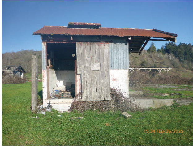
Figure D-10. Area 2 shed view from the exterior.
