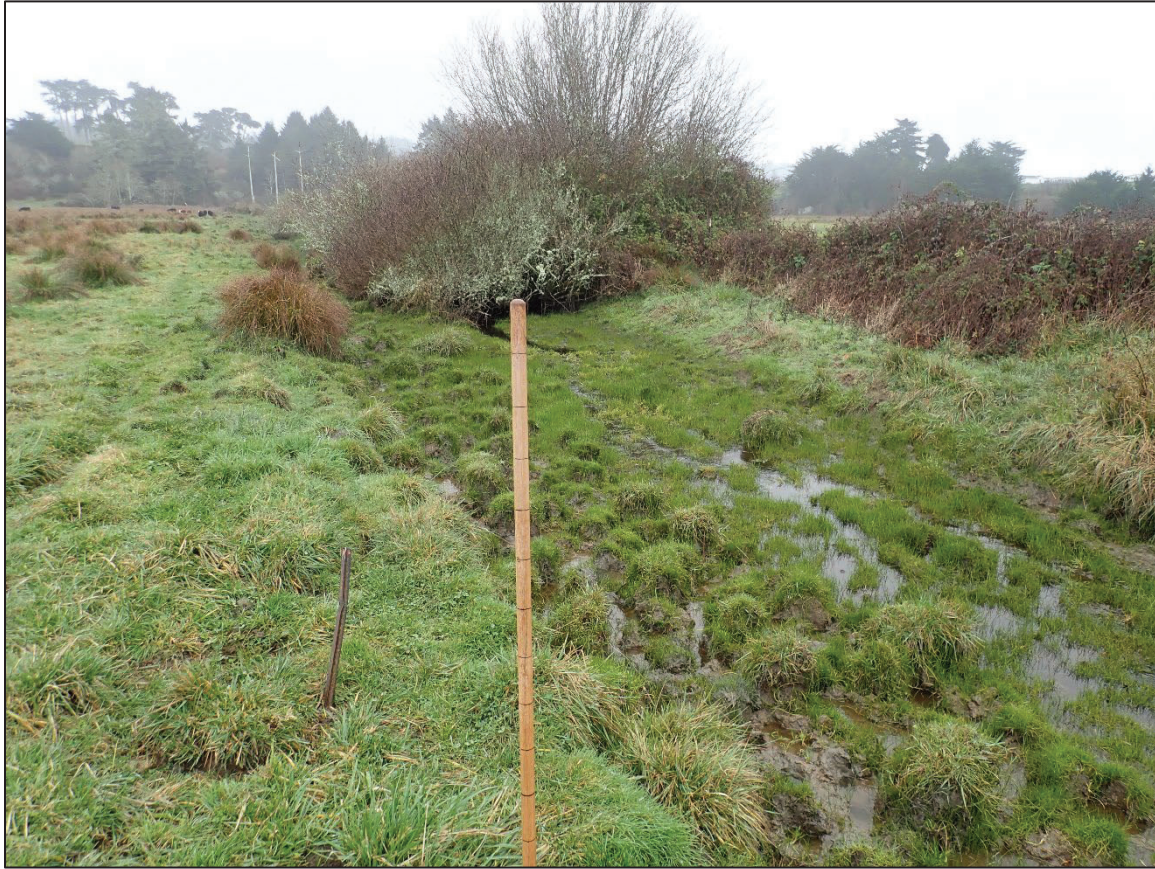
Figure C-6. Photo from January 2022 showing the lower portion of the drainage ditch at ER9.1.
