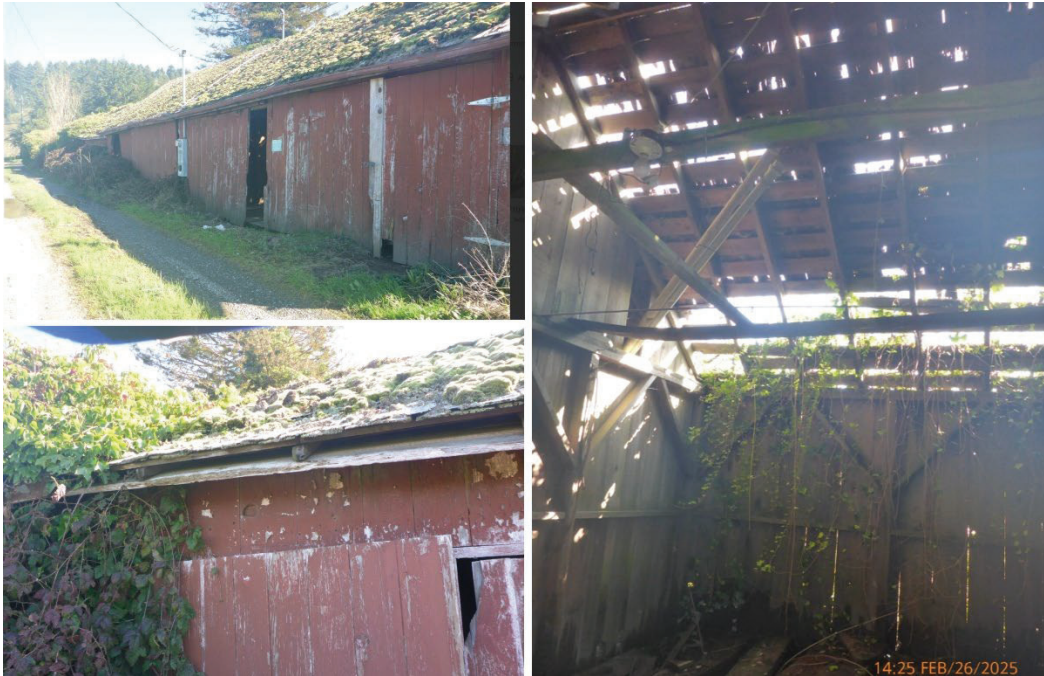
Figure D-5. Area 1 red shed exterior view (top left), view of the interior (right), and potential bat roosting habitat at the roof (bottom left).
