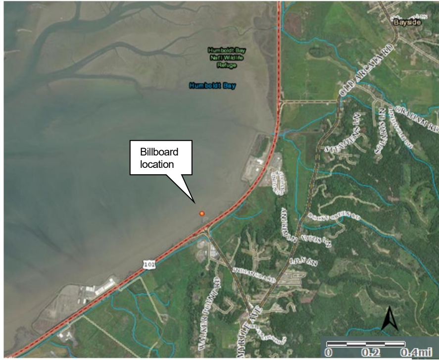
Figure 2: Location of Billboard Repair Project
