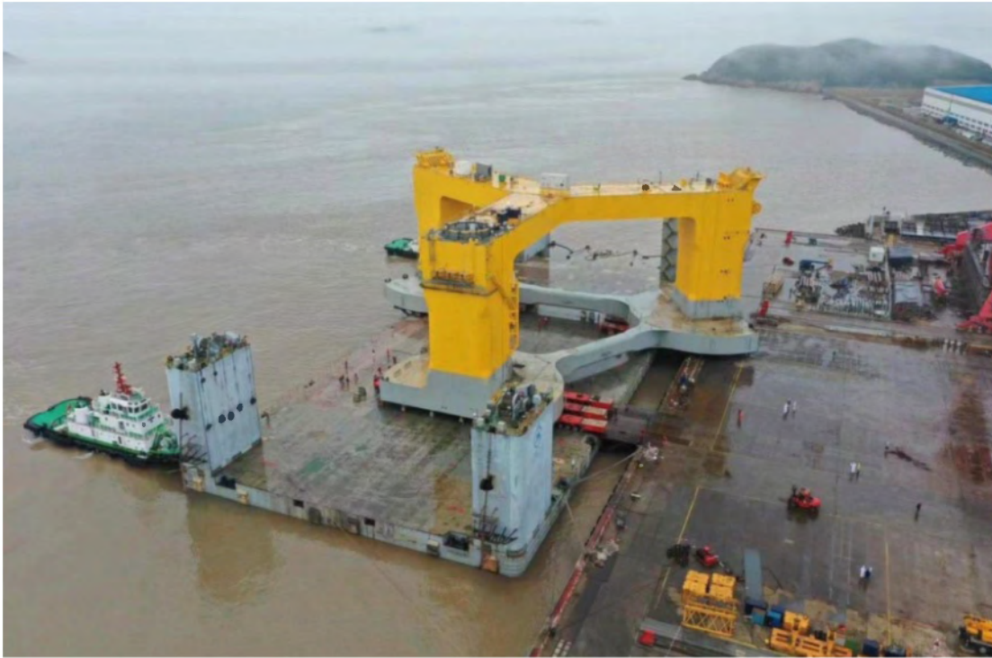
FIGURE 4-1: SEMI-SUBMERSIBLE FOUNDATION BEING LOADED ONTO A SEMI-SUBMERSIBLE BARGE USING SPMTS (Source: Wilson Offshore & Marine)
