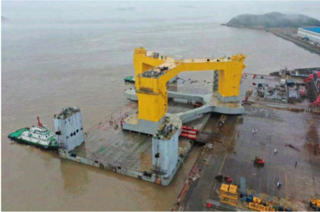
FIGURE 4-1: SEMI-SUBMERSIBLE FOUNDATION BEING LOADED ONTO A SEMI-SUBMERSIBLE BARGE USING SPMTS (Source: Wilson Offshore & Marine)
