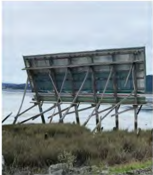
Photo 2. Billboard Unit #4567A initial storm damage
