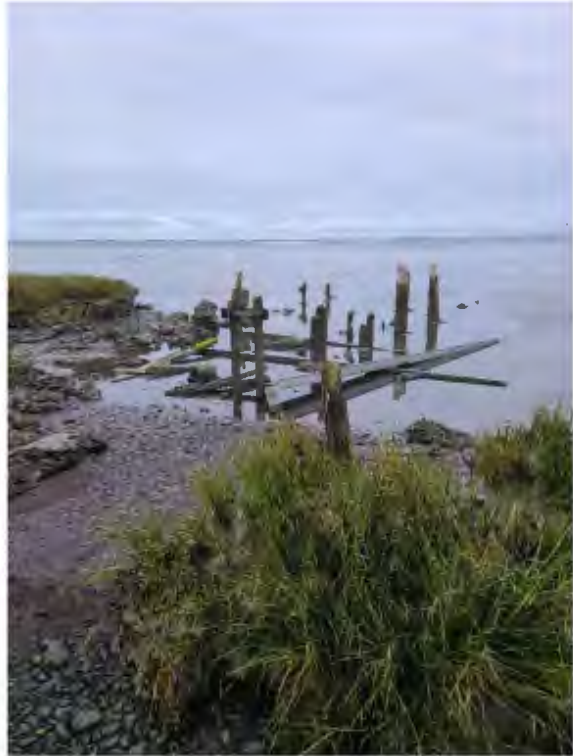
Photo 4. Billboard pilings to be removed & replaced
