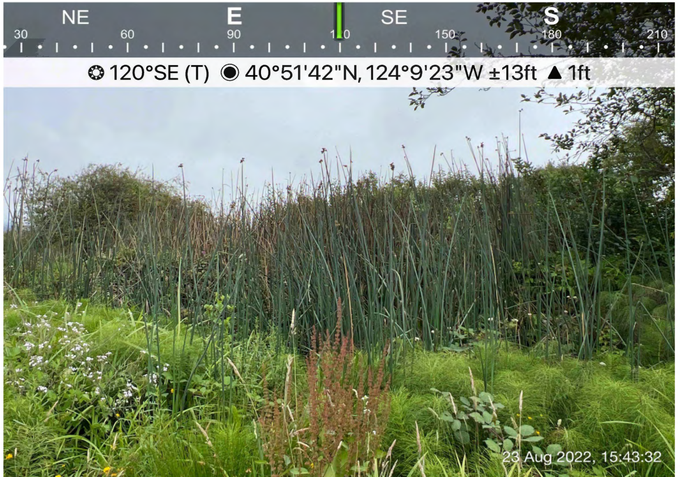
Photo 1 Tall vegetation blocking views towards the culvert replacement.
