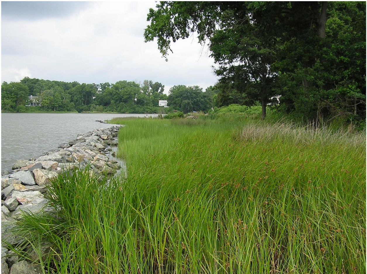
Figure 24: Sill placed in front of an eroding shoreline 31
