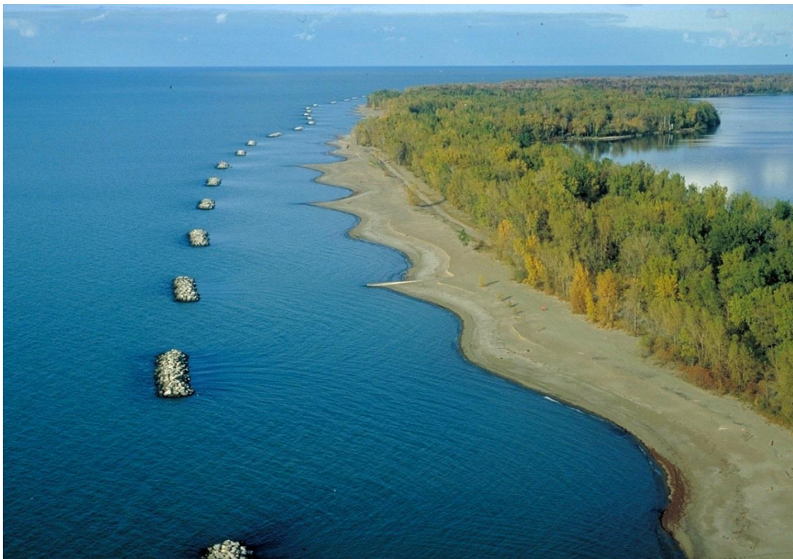
Figure 22: Offshore breakwaters in Presque Isle, PA 28
