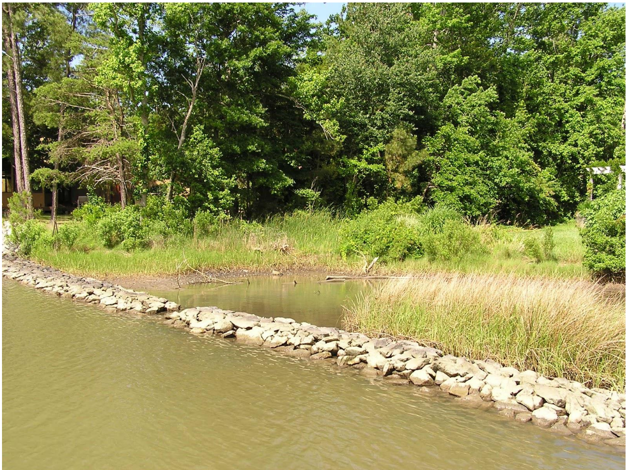
Figure 25: Marsh toe revetment 33
