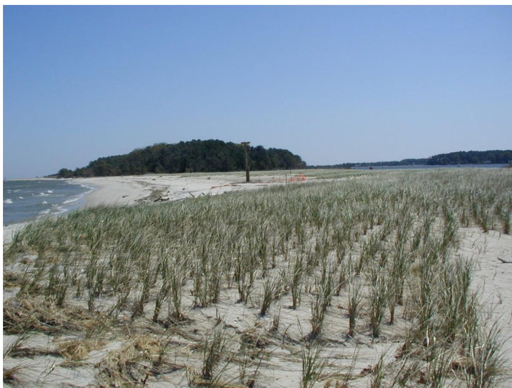
Figure 11: Dredged material placed on a pre-existing shoreline that experienced heavy erosion and then replanted with American beach grass along the Potomac River 7
