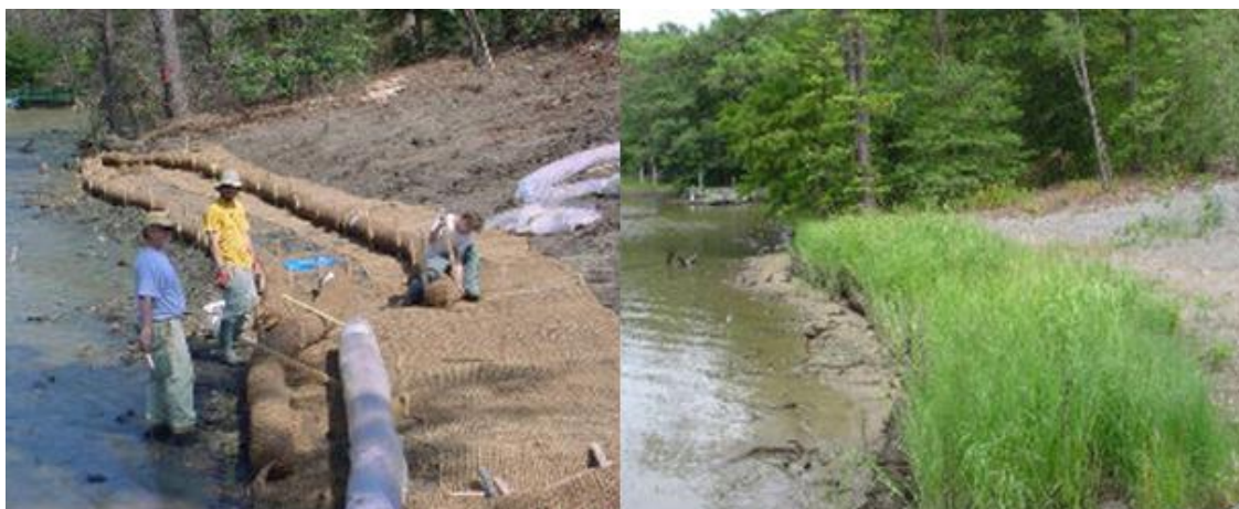
Figure 9: Before and after photos of a natural fiber log embankment project 3
