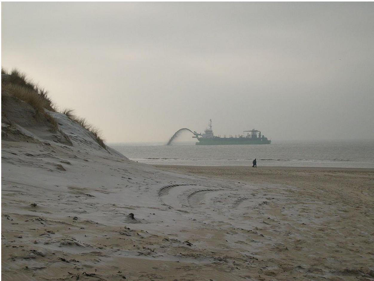
Figure 10: Beach nourishment in the Netherlands. Sand is brought in and dumped near shore to let natural currents refresh the sands along the coastline 5
