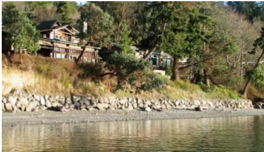
Figure 16: Toe revetment placed at the base of an eroding bank, uses established vegetation 17
