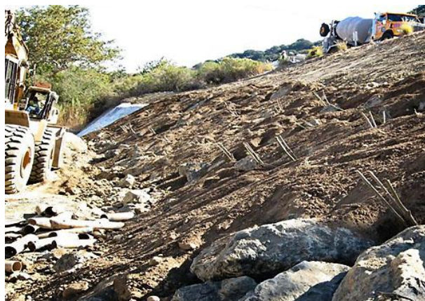
Figure 21: Caltrans backfilling soil over RSP before planting vegetation on the slope 27
