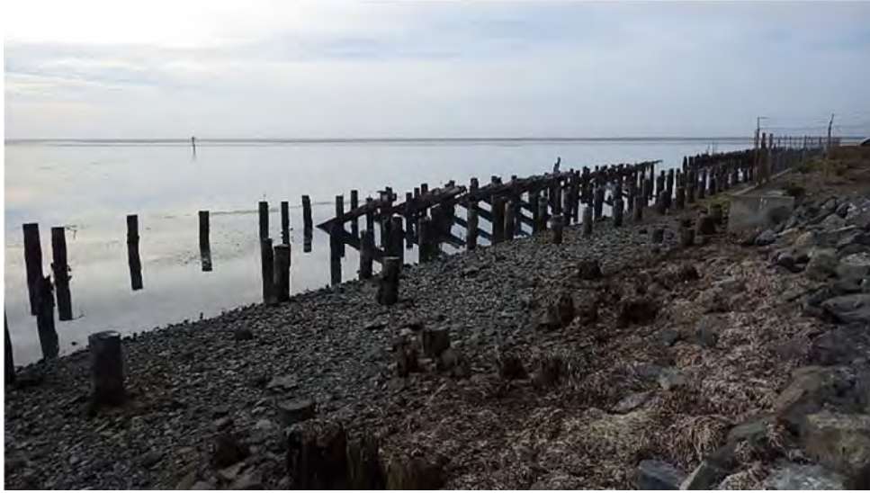
Figure 10. Dilapidated pilings and cobble/gravel fill at the Fields Landing eelgrass mitigation site.
