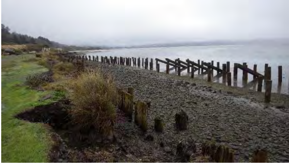
Figure 6. Eroding shoreline, remnant pilings, and gravel/cobble fill in the mitigation area.
