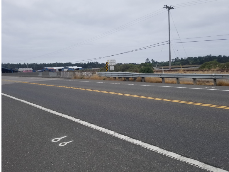
View of south Side of the Mad River Slough looking west towards the Sierra Pacific Saw Mill
