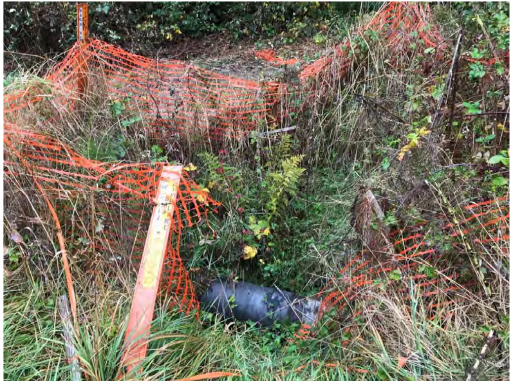
Photograph O. Northwest view of exposed pipeline in sinkhole at RT- 102 Site. Photograph taken 10/31/18.
