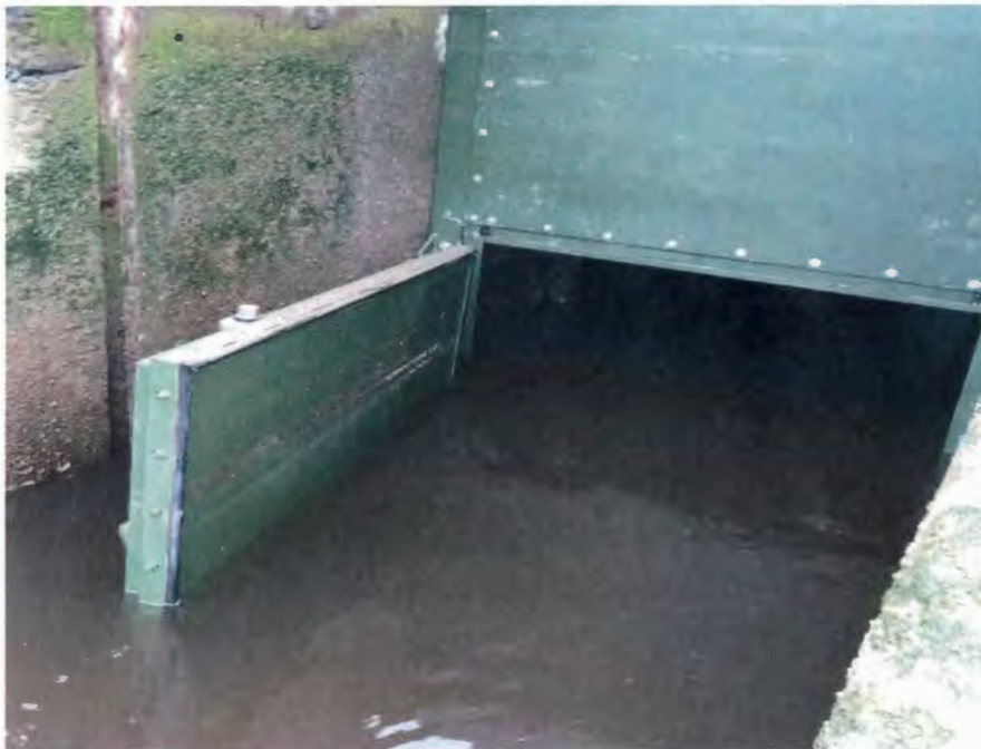
Post-Construction: New 5' x 5' side hinge gate installed and operating on an outgoing tide.
