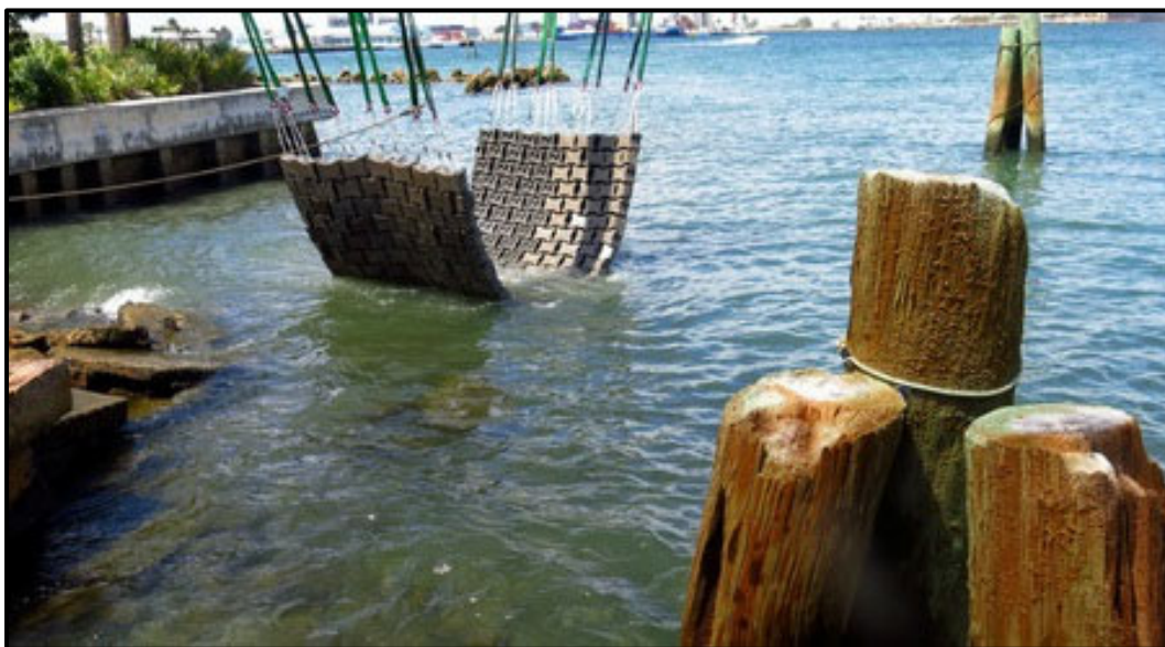
Figure 2.1-5. Shoreline Stabilization Mat (Example)
