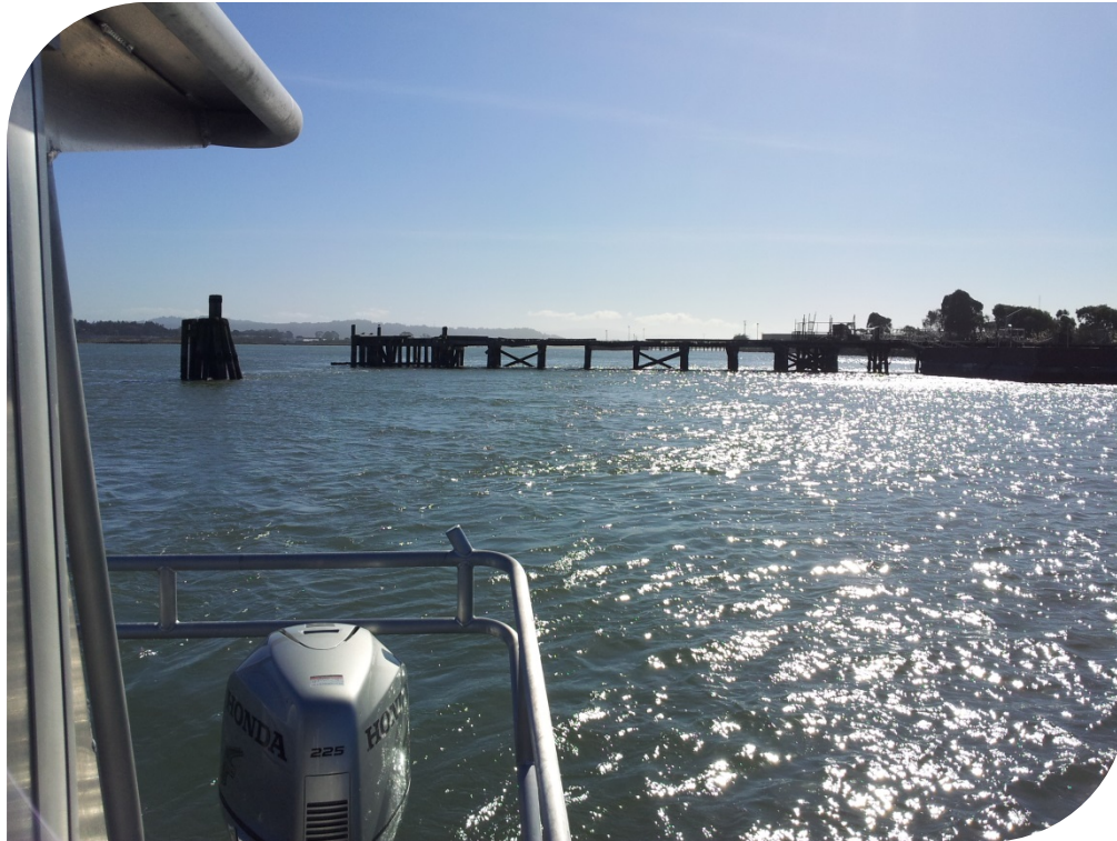
Photo 7 — Pier, from north.
