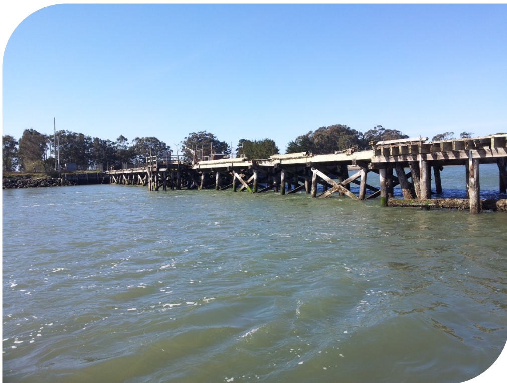
Photo 8— Pier, from south.
