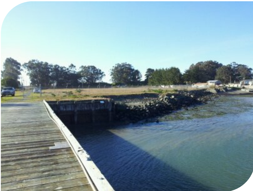
Photo 6 — View of riprap shoreline, from pier.
