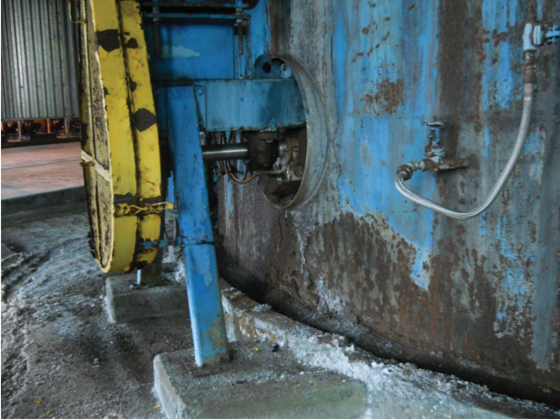
Oxidation of metal and ubiquitous mineralization of surfaces on ground floor of Recovery Boiler #3.
