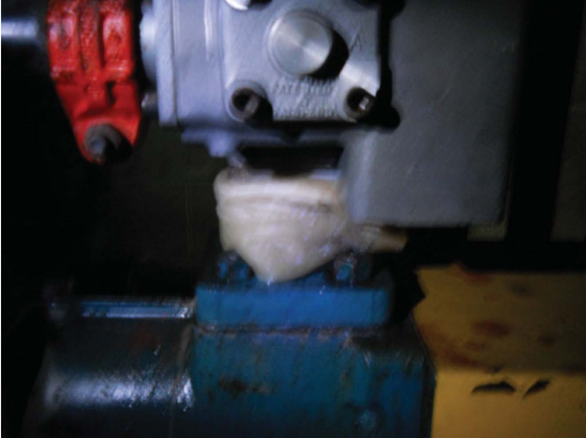
Adsorbent pad on hydraulic pump for Offices/Shops/Stores building elevator. Darkness was a limiting factor in this room.
