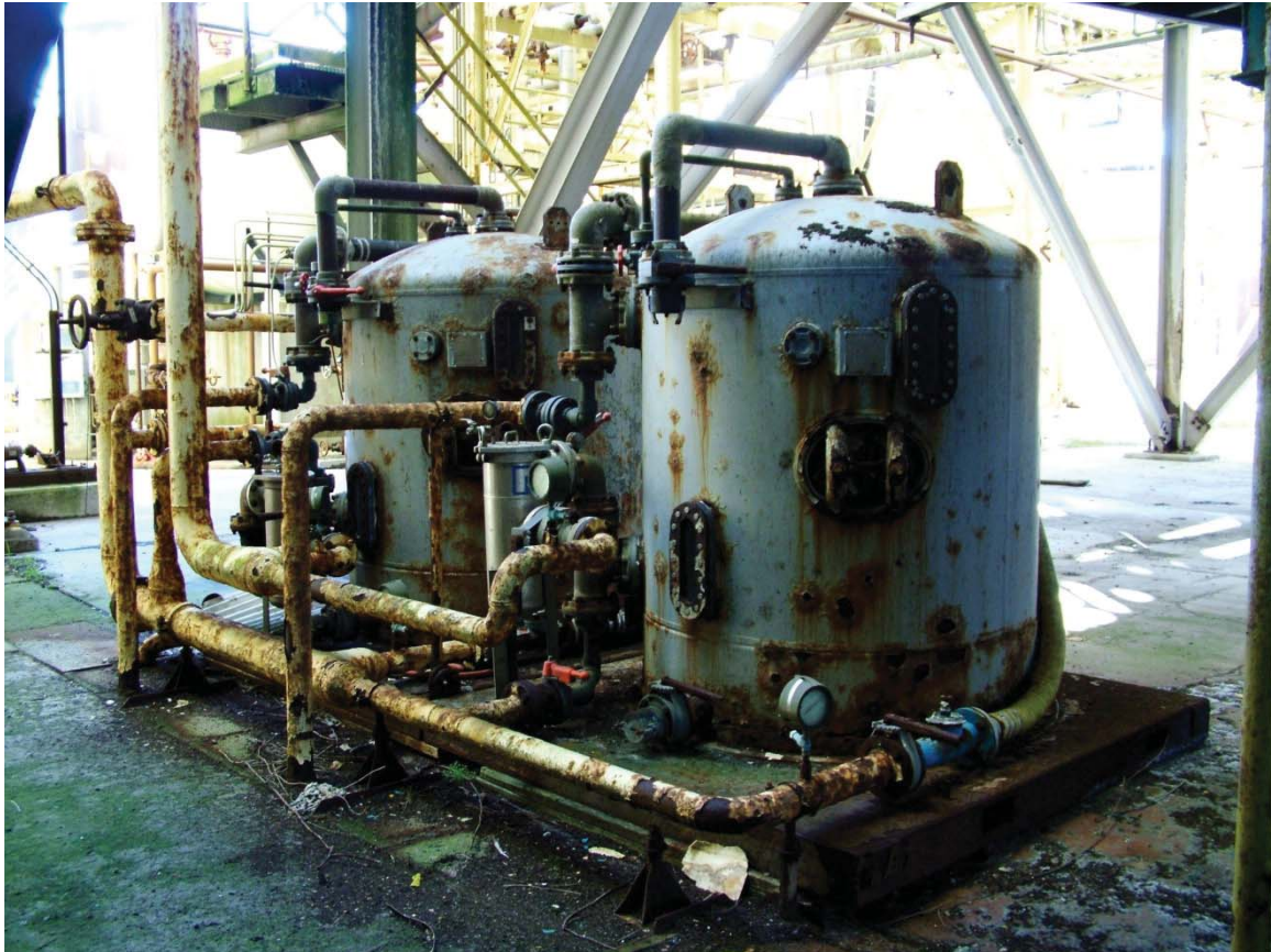
Corrosion of metal surfaces and concrete in AOI-1 Black Liquor Process and Recovery Area.
