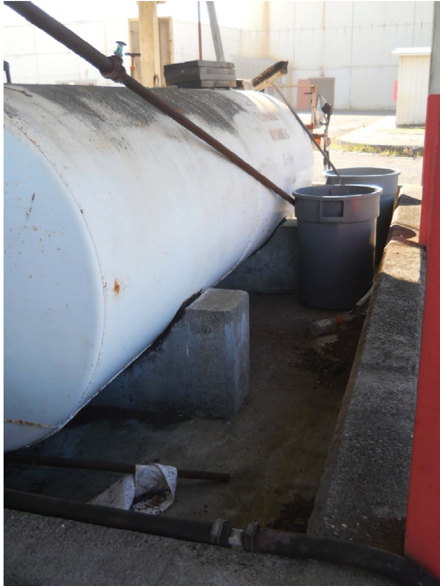
1,000-gallon Unleaded gasoline AST in secondary containment at AOI-10 Petroleum Hydrocarbon Storage Area. Photograph taken facing southwesterly.
