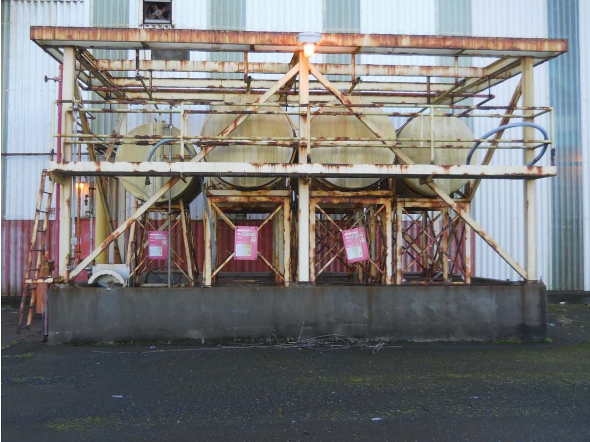
ASTs on racks in a secondary containment located on the northern side of Recovery Boiler #3.
