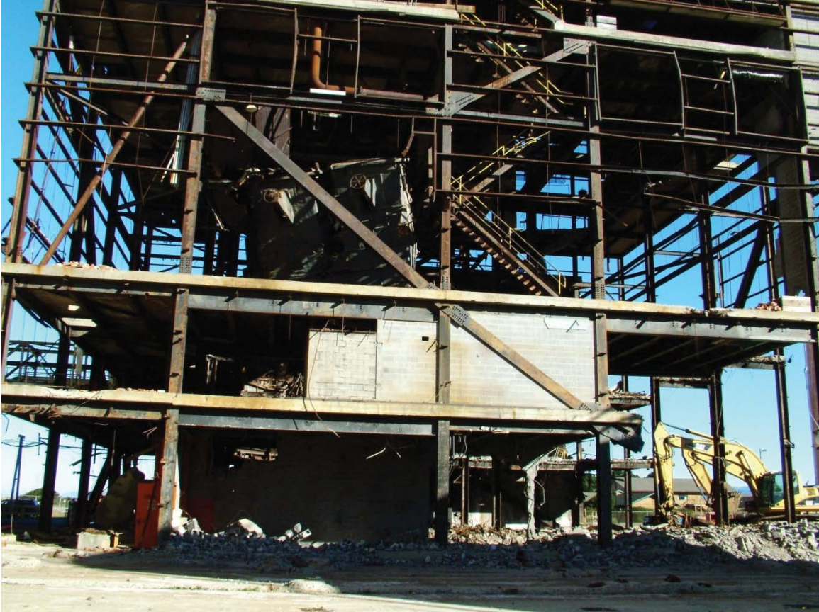
Ongoing demolition of Recovery Boilers 1 and 2 in AOI-1 Black Liquor Process and Recovery Area. Photograph taken facing northerly.
