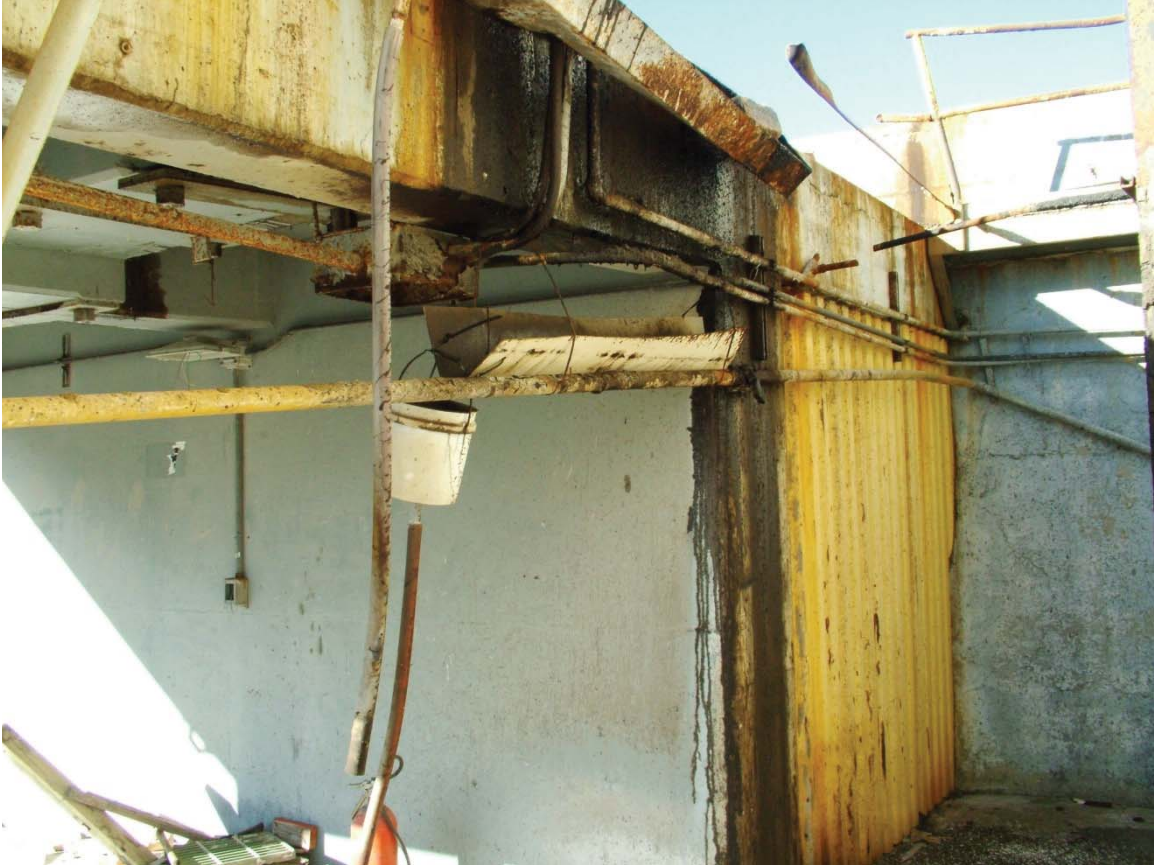
Oil staining on the concrete roof of a shed in the Recausticizing Area. Note attempt at containing the oil by placement of a section of roofing gutter beneath spill, directing the fluids to the bucket, and a hose from the bucket to another container (not shown).
