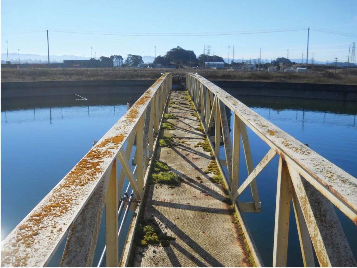
Catwalk extending into the center of a clarifying pond at the Water Treatment Plant.
