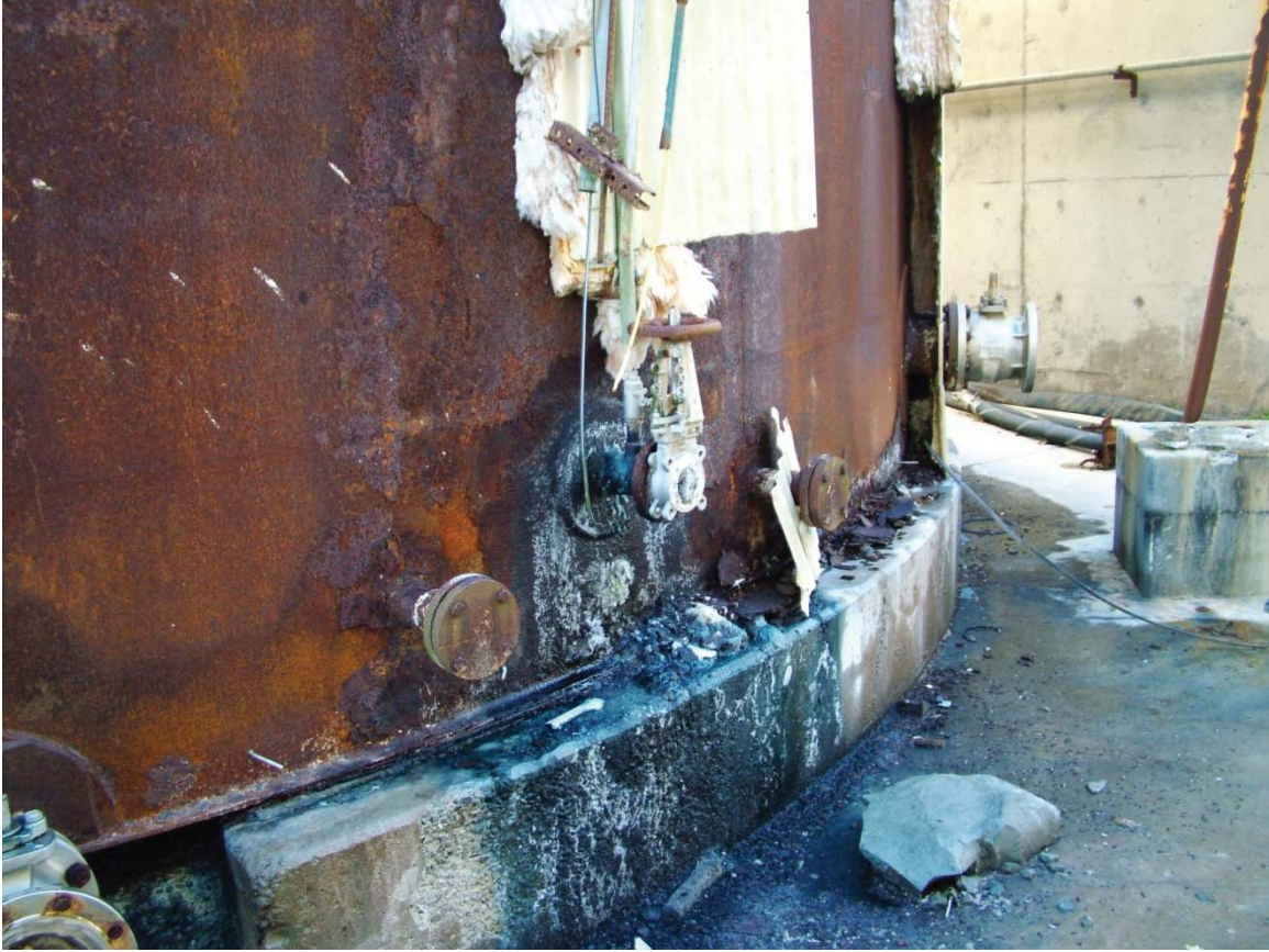
Corrosion, staining and crystal precipitation from an AST in AOI-3, the Recausticizing Area.
