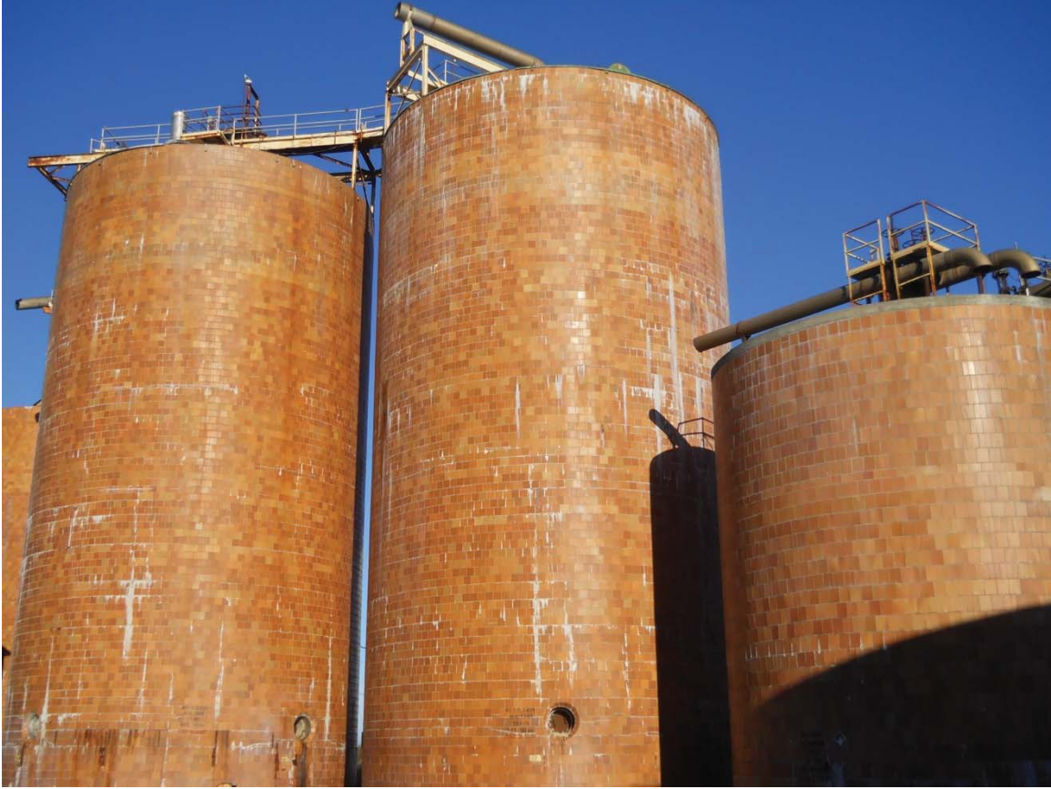
Bleach Plant ASTs used for bleach stock storage. Note discoloration of surfaces indicating leaking occurred. Photograph taken facing southwesterly.
