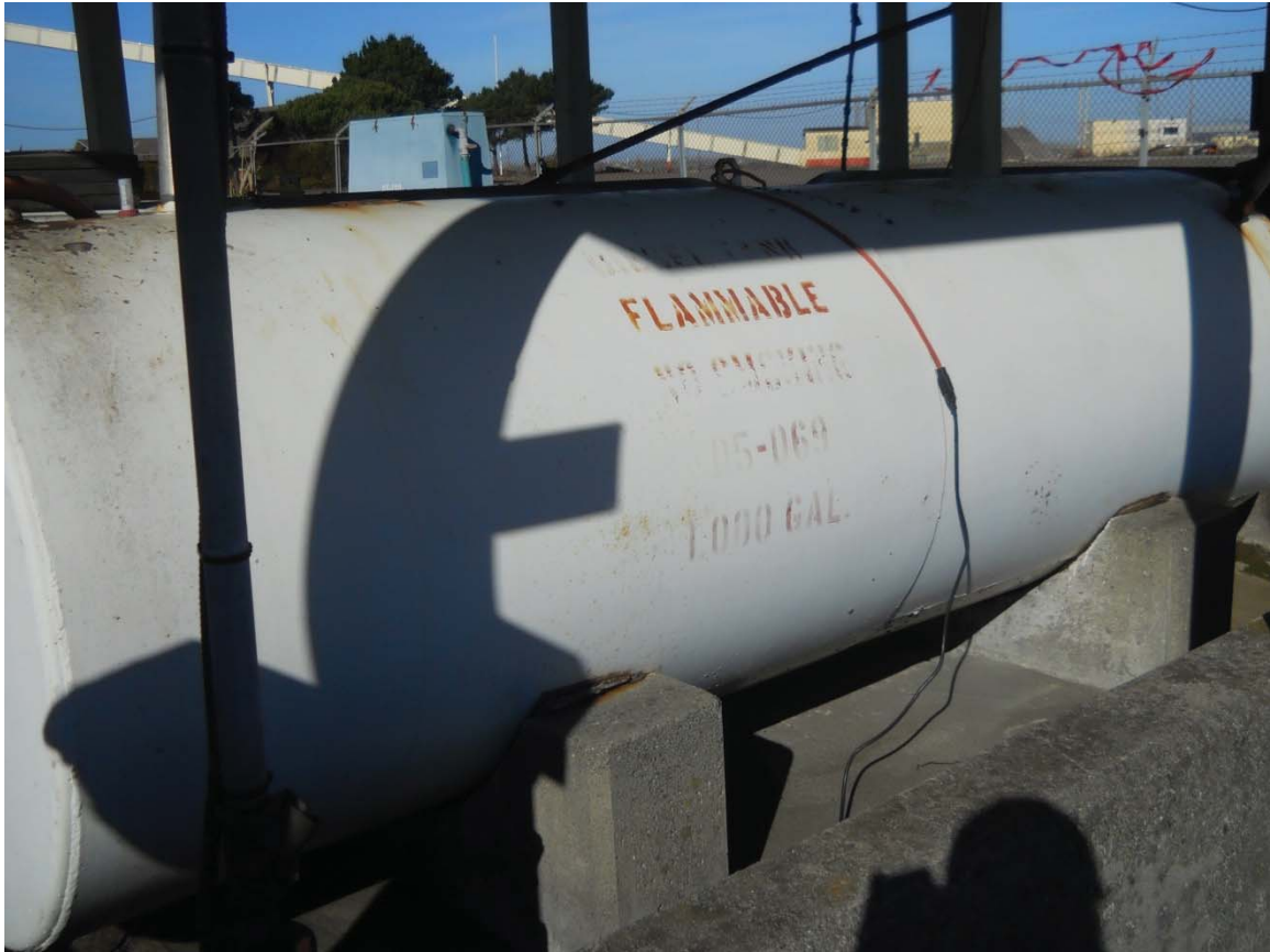
1,000-gallon diesel AST in secondary containment at AOI-10 Petroleum Hydrocarbon Storage Area.
