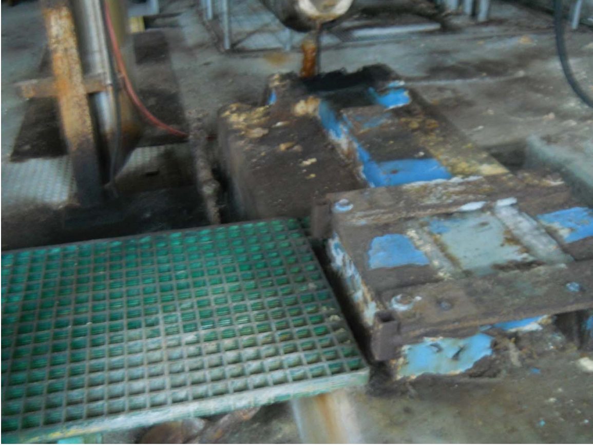
Oxidized and oil-stained motor mount in Recovery Boiler #3.
