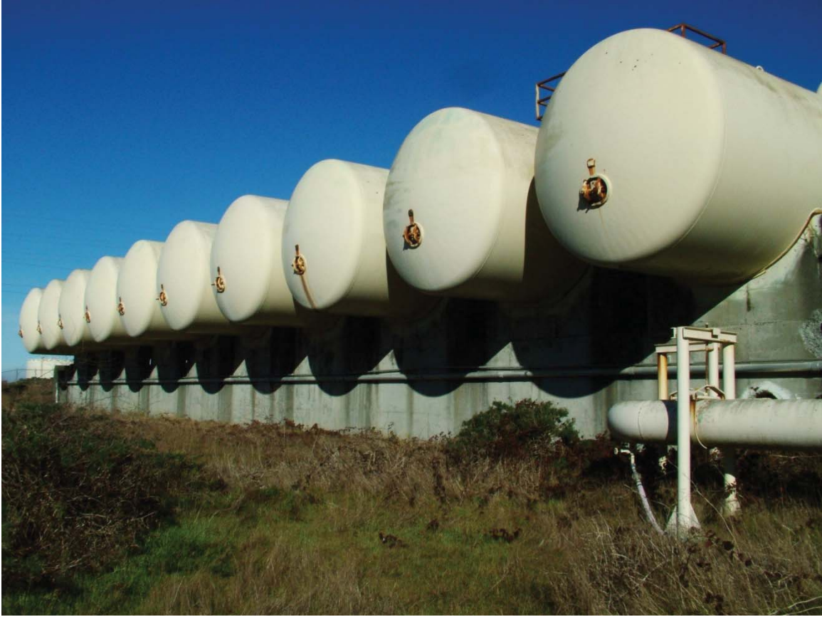
Water Treatment Plant water filters and softeners. Photograph taken facing northwesterly.
