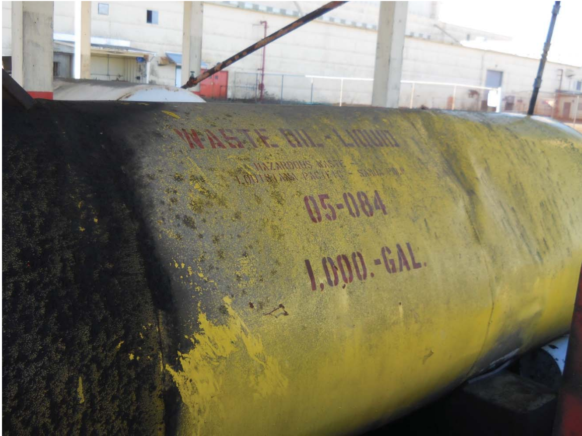
1,000-gallon waste oil AST located at AOI-10 Petroleum Hydrocarbon Storage Area. Note evidence of overflow by the accumulation of oil on exterior of AST. Oil is present on water in the containment, and the fill gauge indicated the presence of oil above the level of the tank (i.e. oil fills the fill tube into the tank).
