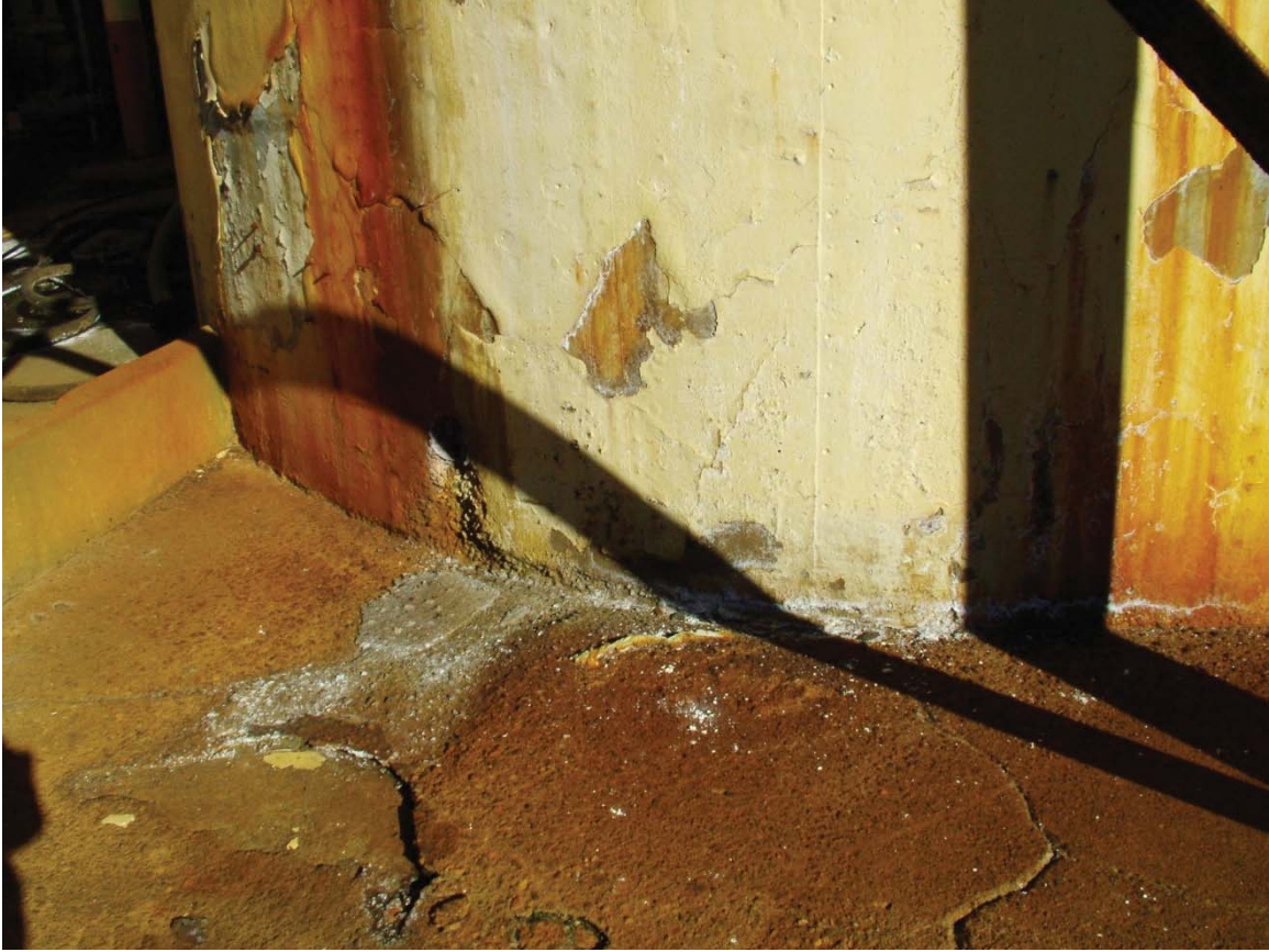
Iron staining and etching of concrete at base of smoke stack in AOI-1 Black Liquor Process and Recovery Area. Photograph taken facing northerly.
