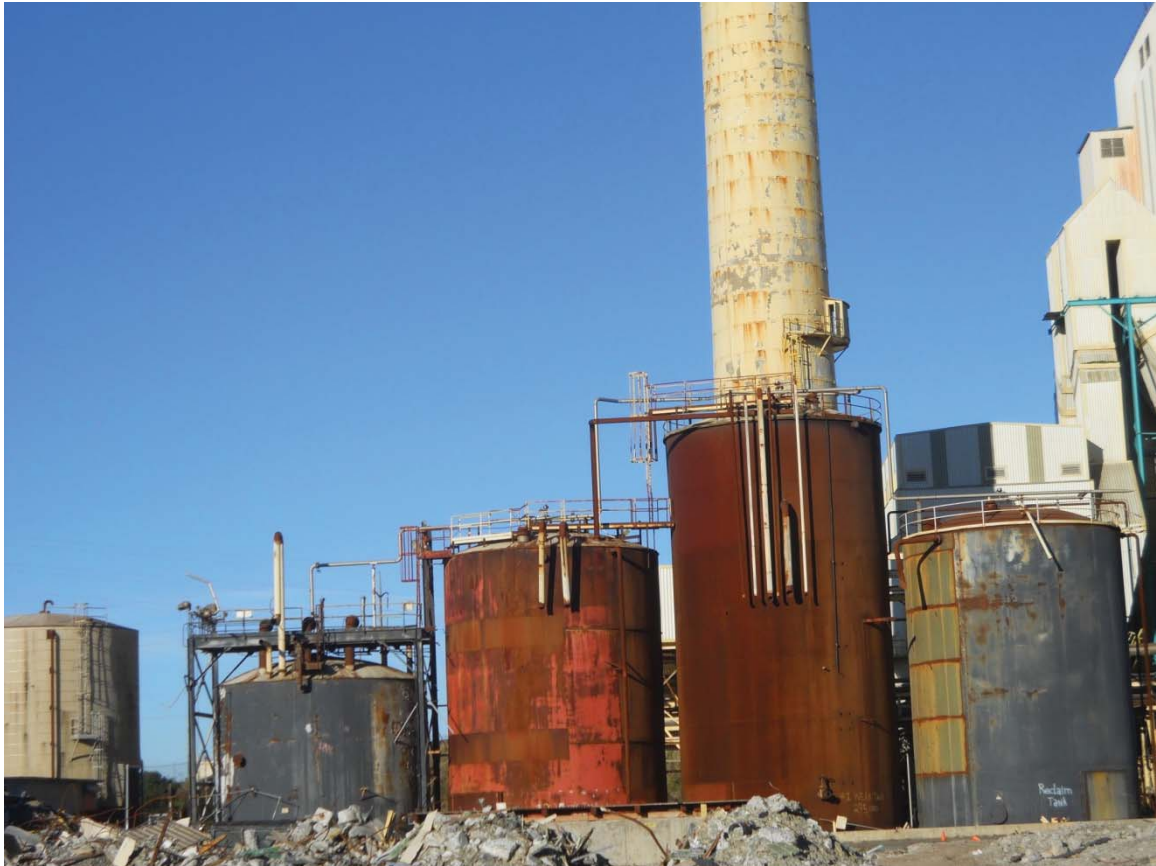
Weak liquor storage ASTs in AOI-1 Black Liquor Process and Recovery Area. Photograph taken facing northerly.
