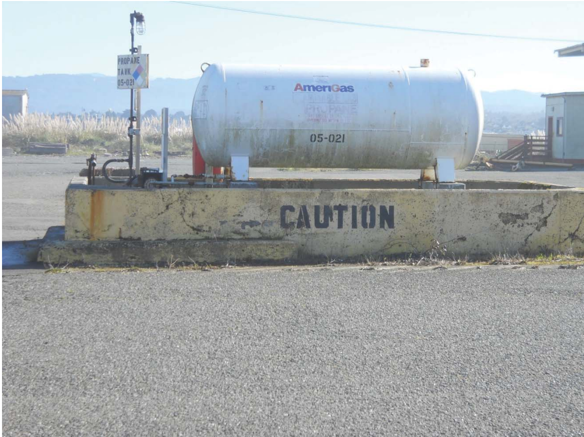
Propane tank in a secondary containment located northerly of Warehouse 1. Photograph taken facing southeasterly.
