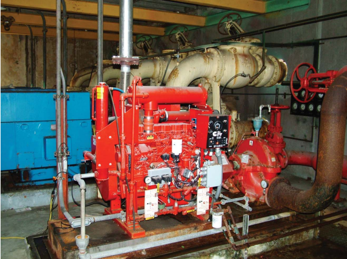
Generator in Pump House in AOI-3. Product distribution lines extend from the 250-gallon AST to the generator, and the lines are rusted.
