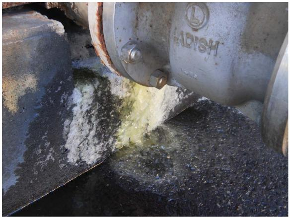
Close up of mineralization of the concrete surface beneath the AST. A strong sulfur odor was present in this area.
