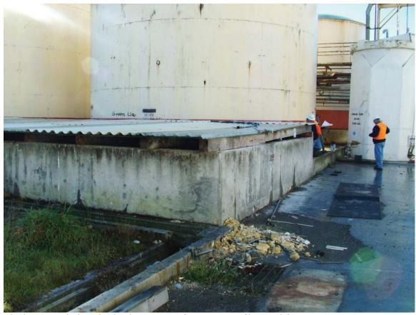
Black Liquor sludge shed adjacent to AOI-5 Process Chemical Storage Area. Note staining of containment walls resulting from sludge leaking through cracks. Photograph taken facing southerly.
