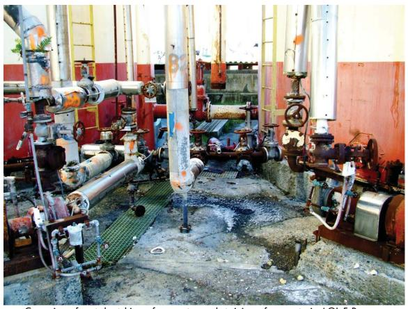
Corrosion of metal, etching of concrete, and staining of concrete in AOI-5 Process Chemical Storage Area.
