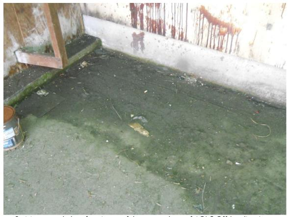
Staining on asphalt surface in one of the storage bays of AOI-9 Off-Loading Area. Source of staining unknown. A rusty one-gallon bucket of latex paint is present in the foreground.
