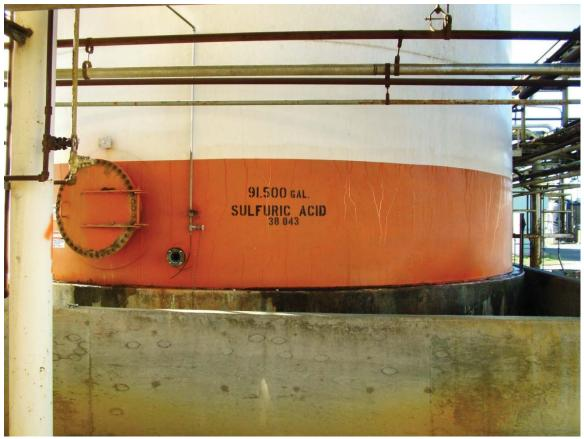
AOI-5 Process Chemical Storage Area Sulfuric Acid above ground storage tank in secondary containment. Photograph oriented facing southerly.
