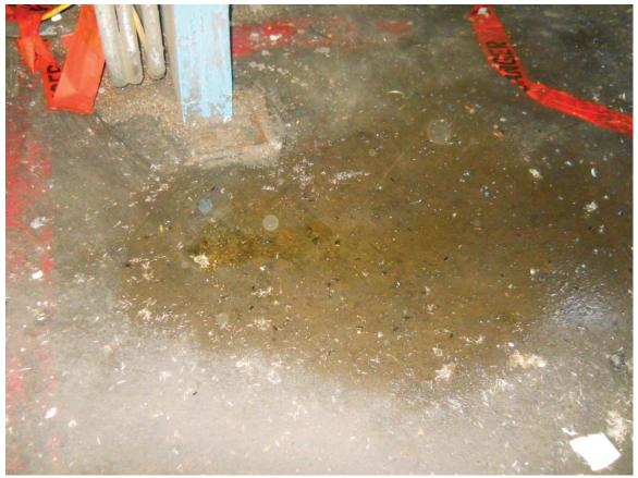
Staining of concrete by hydraulic fluids adjacent to hydraulic presses identified in the previous photographs.
