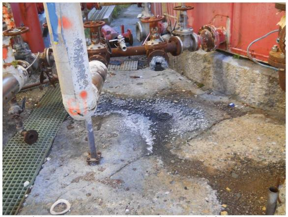
Valve failure, corrosion of metal, and etching of concrete in AOI-3, the Recausticizing Area.
