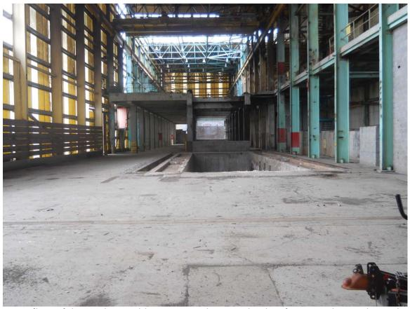
First floor of the Machine Building interior. Photograph taken facing northwesterly. Pool for collection of liquids during pulp compression in mid-ground.
