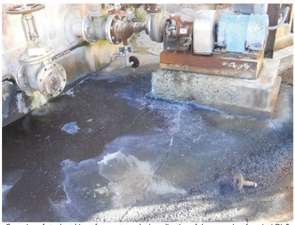
Corrosion of steel, etching of concrete and mineralization of the ground surface in AOI-5
