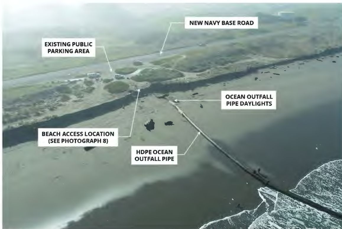
Photograph 7. Beach and outfall pipe access location. View looking south-southeast. Taken March 14, 2024, 10:10 AM. Approximate tide level -0.33 feet, NAVD88.
