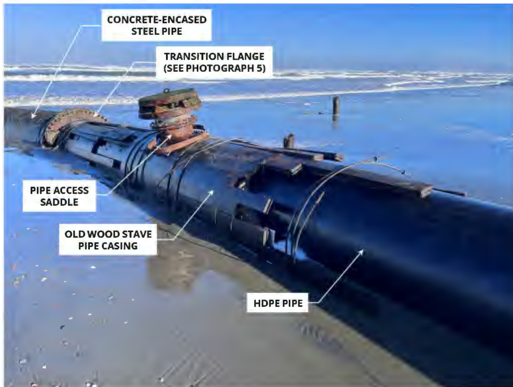
Photograph 4. Ocean outfall pipe transition zone from HDPE pipe to concrete-encased steel pipe. View looking west-northwest. Taken March 14, 2024, 9:10 AM. Approximate tide level -0.15 feet, NAVD88.
