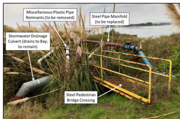
Image 1: Existing stormwater feature to be replaced
