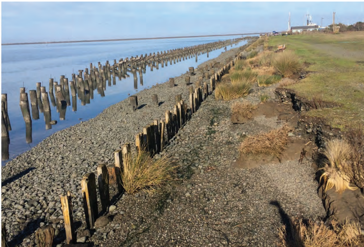
Figure 2. Photo of representative shoreline erosion at project site. Photo source: Stillwater Sciences, 2016
