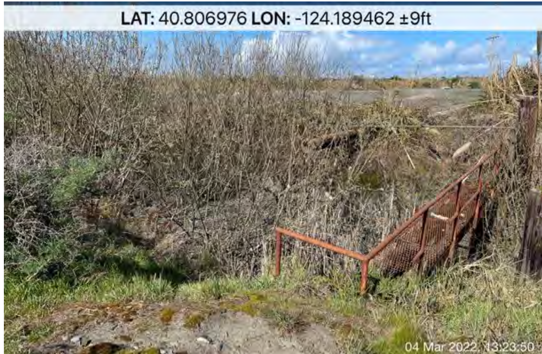
Photo 6: Stormwater swale showing one of three pedestrian bridges looking north. Note edge of willow canopy at bridge signifying the edge of ESHA. Photo taken March 4, 2022.
