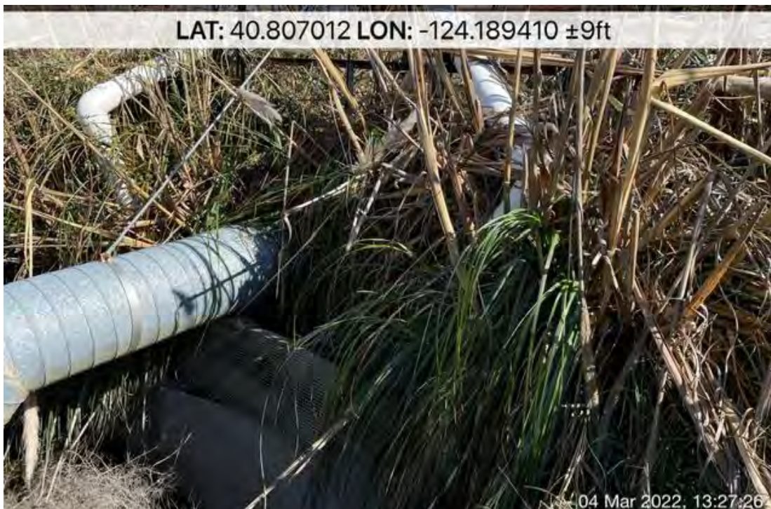
Photo 8: Closeup at existing stormwater detention infrastructure. Note weirs, screening, and overflow pipes. Photo taken March 4, 2022.
