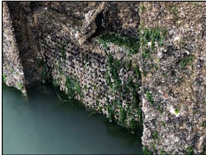
Image 4: Existing water intake screen at the Redwood Marine Terminal II Dock. This screen will be replaced.
