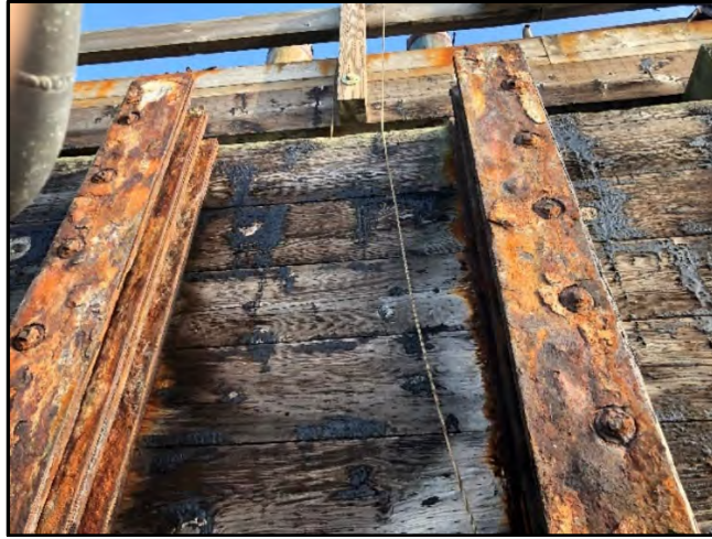
Image 3: Existing wooden sea chest at the Redwood Marine Terminal II Dock. This sea chest will continue to be utilized.
