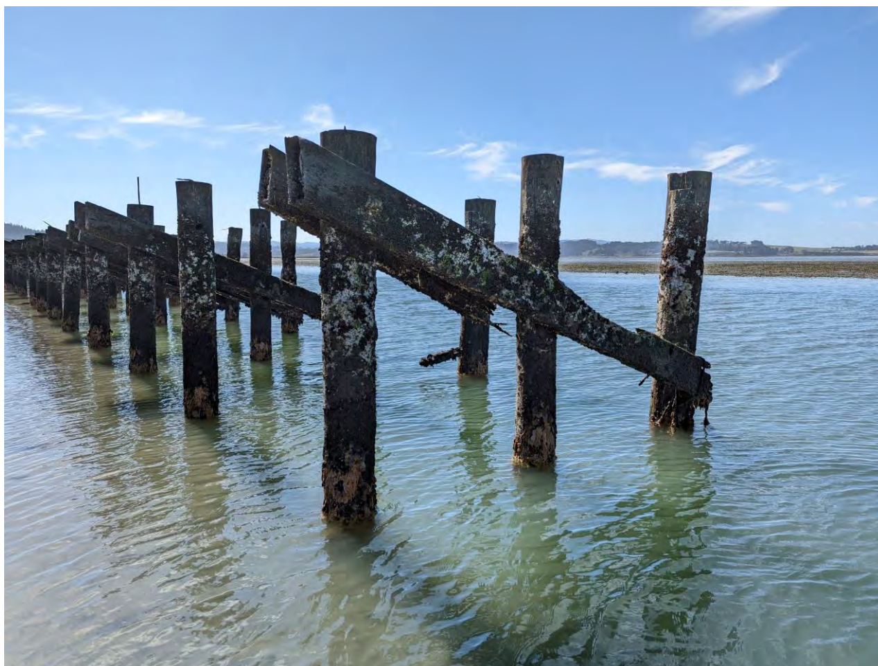
Figure 1 Typical piles and cross beams at mitigation site.
