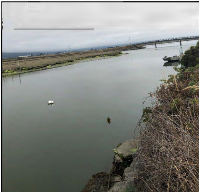
Lanphere Road bridge in background and project site in foreground.
