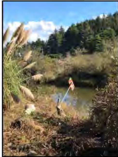
Figure 2.2-2. R-519 Retired Pipeline Crossing Across Ryan Slough
