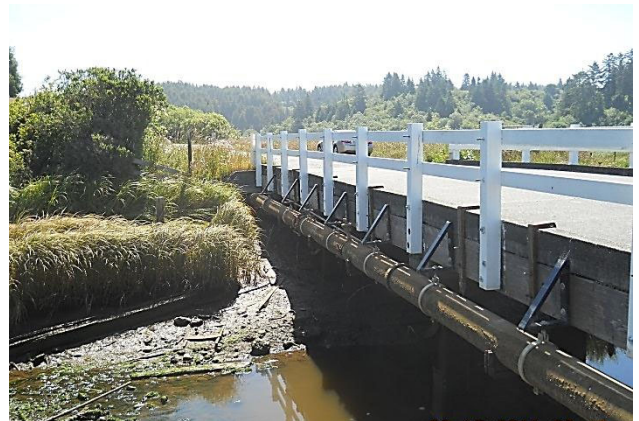
Figure 3: Existing Water Line
