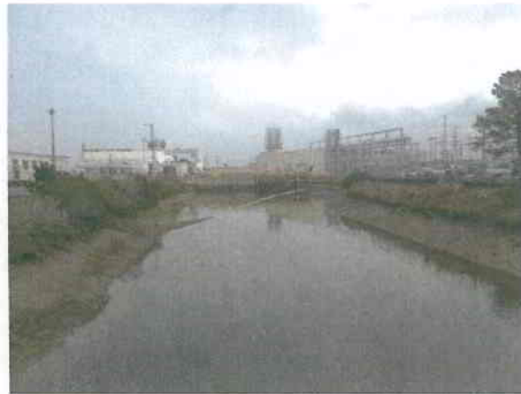
FIGURE 5 The Intake Canal Between the Pedestrian Bridge and the Intake Structure
